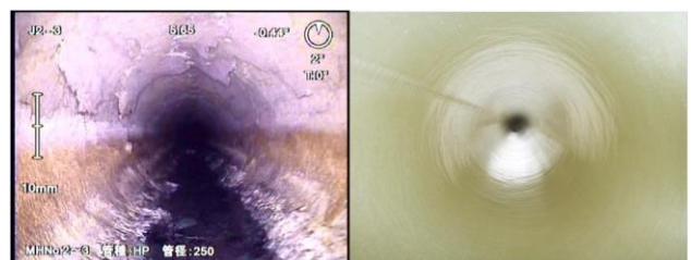
Fig. 10 Pipeline renovation before (left) and after (right) using our glass cylindrical material with resin-impregnated composites.
